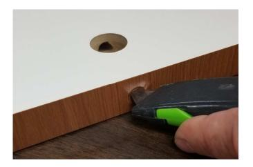
d) CUT OUT FOIL COVERING ELONGATED SLOT ON JOINING END OF TOPS (requires utility knife)
