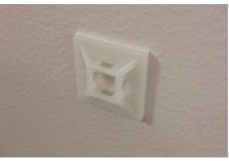
b) SLIDE TIE THROUGH WALL HOLDER – WITH CONNECTOR TO OUTSIDE
