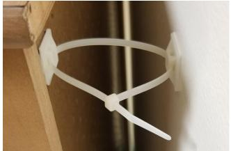
e) TIGHTEN TIE TO DESIRED DEPTH FROM WALL – CUT OFF EXCESS
